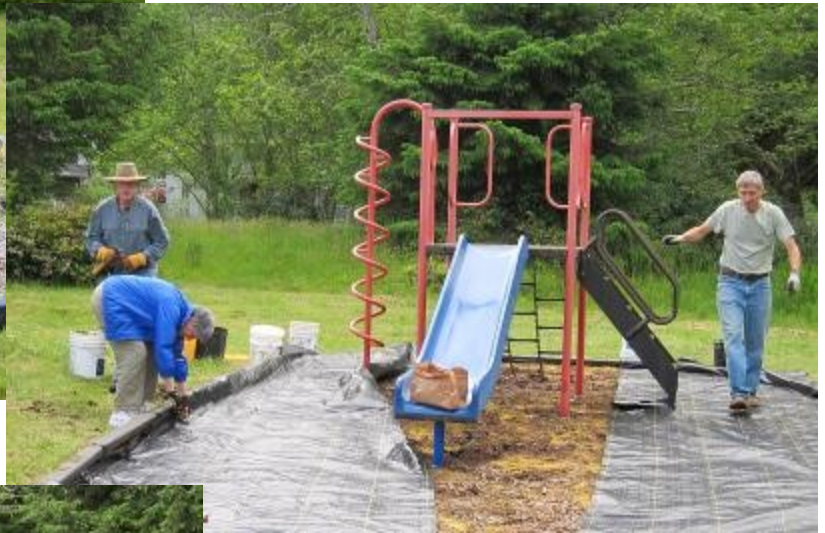
Laying Ground Cloth
